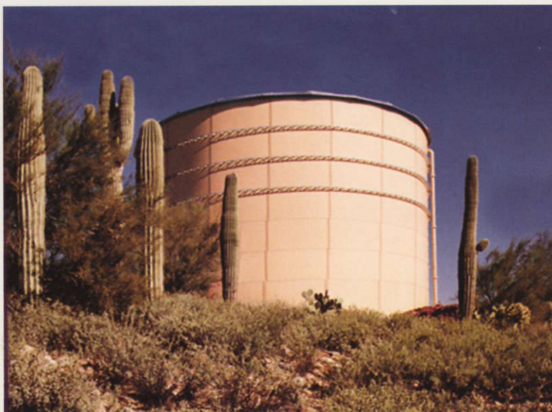
Aquastore's glass coatings meet ANSI/NSF Standard 61 requirements for indirect additives, making them suitable for potable water storage.
